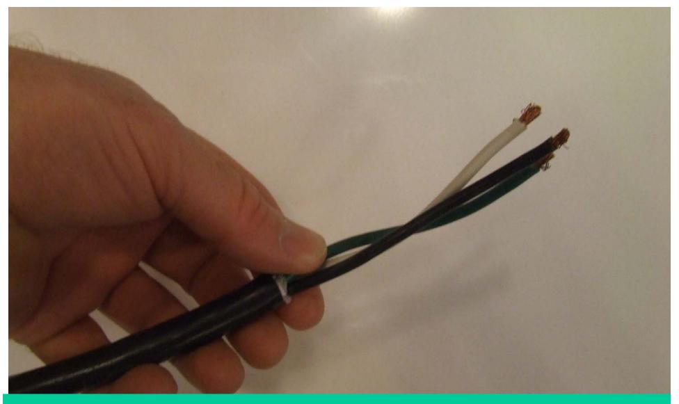
The factory supplied plug is cut off, the insulation is stripped back and the insulation on the conductors is also stripped back
