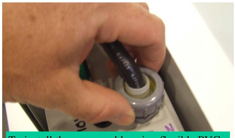
To install the power cable using flexible PVC conduit, remove the threaded compression nut from the Liquid Tight coupler
