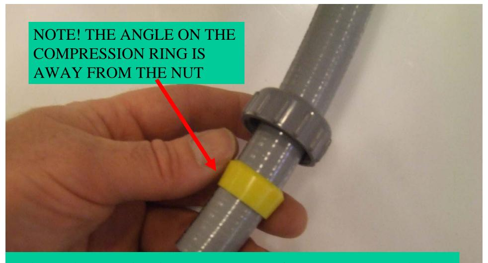
The threaded compression nut and the compression ring are slipped over the conduit
